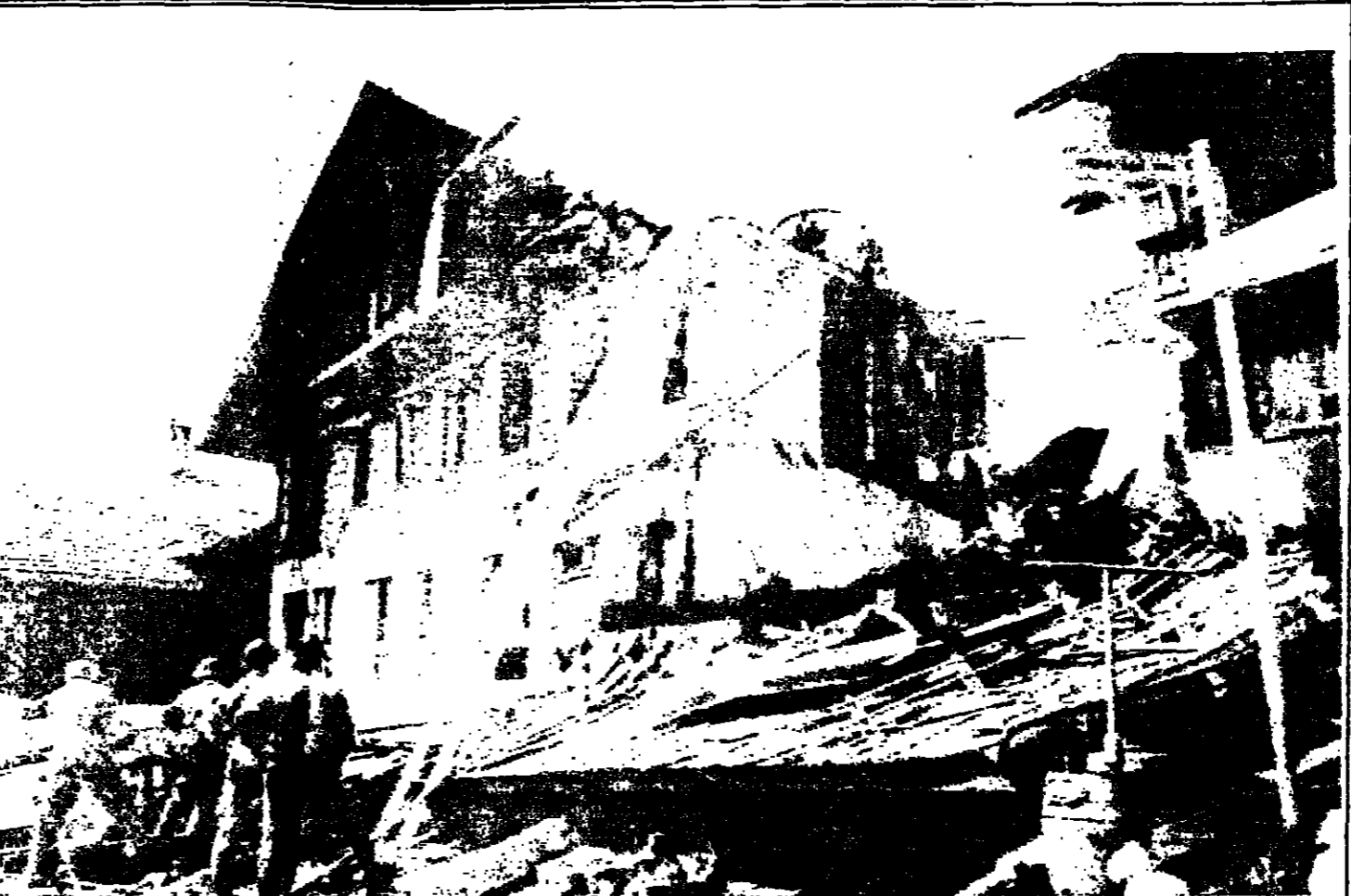
WRECKAGE: This is what remained of a house at Zweismen, Bernes Overlands, when a Mirage aircraft of the Swiss Air Force crashed into the building after a collision with a Tiger F5E Thursday morning. One person was killed in the house. The Tiger Jet crashed near Adelboden. Both pilots sustained injuries.
